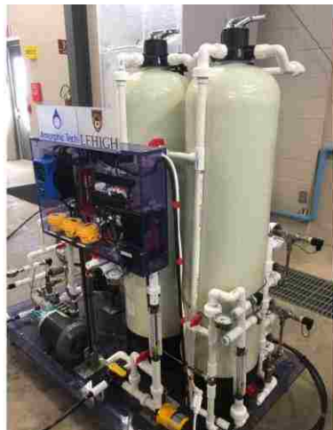
Figure 6-3. Pilot test in BNGDRF, Alamogordo, NM.
